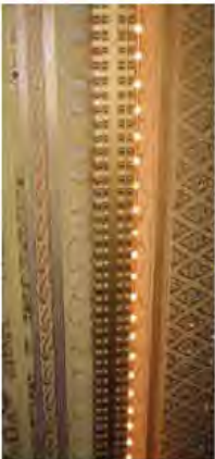
Recommended: [62-63] Carefully installed new mechanical ductwork is barely visible in the elaborately decorated ceiling of this historic theater. [64] The ductwork has been left unpainted which is compatible with this historic industrial interior. [65] To avoid damaging the metal ceiling, the ductwork was left exposed and it was painted to minimize its impact, thus preserving the historic character of this former bank.
