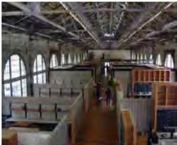
Recommended: [62-63] Carefully installed new mechanical ductwork is barely visible in the elaborately decorated ceiling of this historic theater. [64] The ductwork has been left unpainted which is compatible with this historic industrial interior. [65] To avoid damaging the metal ceiling, the ductwork was left exposed and it was painted to minimize its impact, thus preserving the historic character of this former bank.
