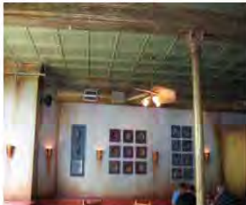
Recommended: [62-63] Carefully installed new mechanical ductwork is barely visible in the elaborately decorated ceiling of this historic theater. [64] The ductwork has been left unpainted which is compatible with this historic industrial interior. [65] To avoid damaging the metal ceiling, the ductwork was left exposed and it was painted to minimize its impact, thus preserving the historic character of this former bank.
