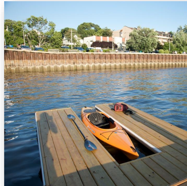
Figure 14: Small boat ramp / dock for non-motorized boats
