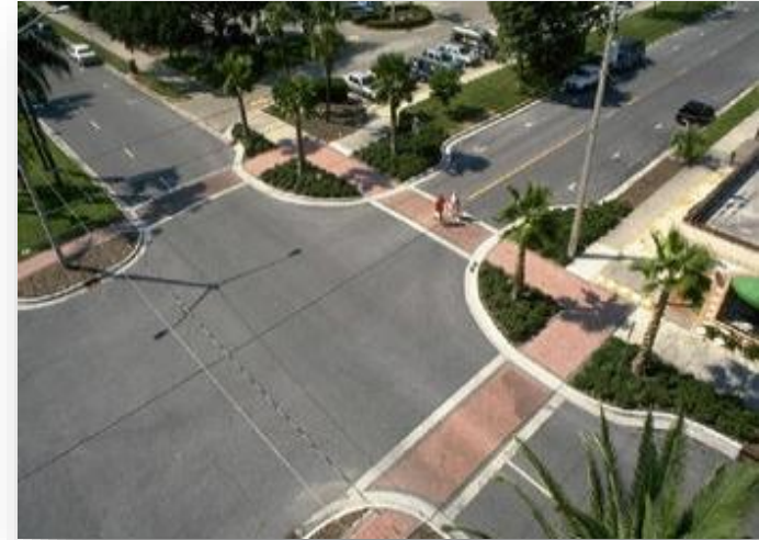
Figure 7: Example of bump outs and curb returns
