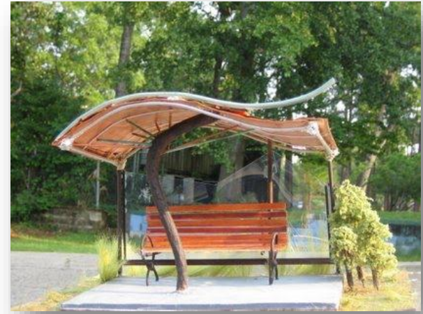
Figure 16: Bus shelter as a significant object in the landscape
