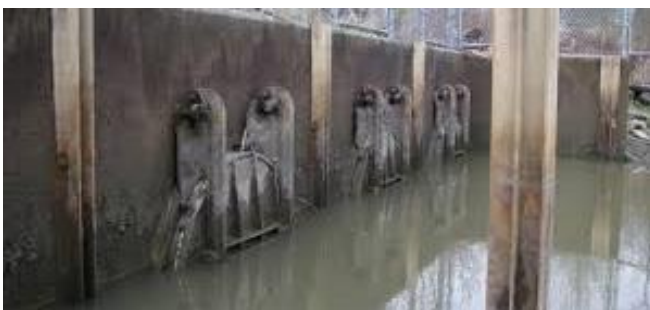
Top mounted floodgates on a tributary of the Lower Fraser River.
